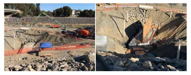
The first of three years of construction is well underway on the major fish ladder project in lower Alameda Creek. This fishway will allow steelhead and salmon to bypass the 12' high BART weir and the adjacent rubber dam. Contractors for ACWD are currently excavating and pouring foundations to anchor the lower end (the entrance) to the eventual fish ladder.
